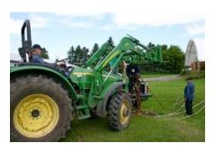
submersible pump at the bottom of the 200 foot well stopped working. This well provides the water for the cows and the milking parlour, so it is an emergency when it does not function. Jim, Ben and Juanito along with our local plumber spent most of the day raising the steel water line and broken pump and replacing it with a plastic line and a new submersible pump. Replacement parts were
